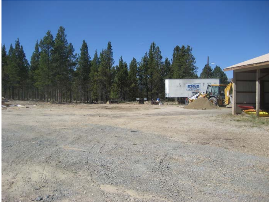
15. ORL Site Facing WEST
